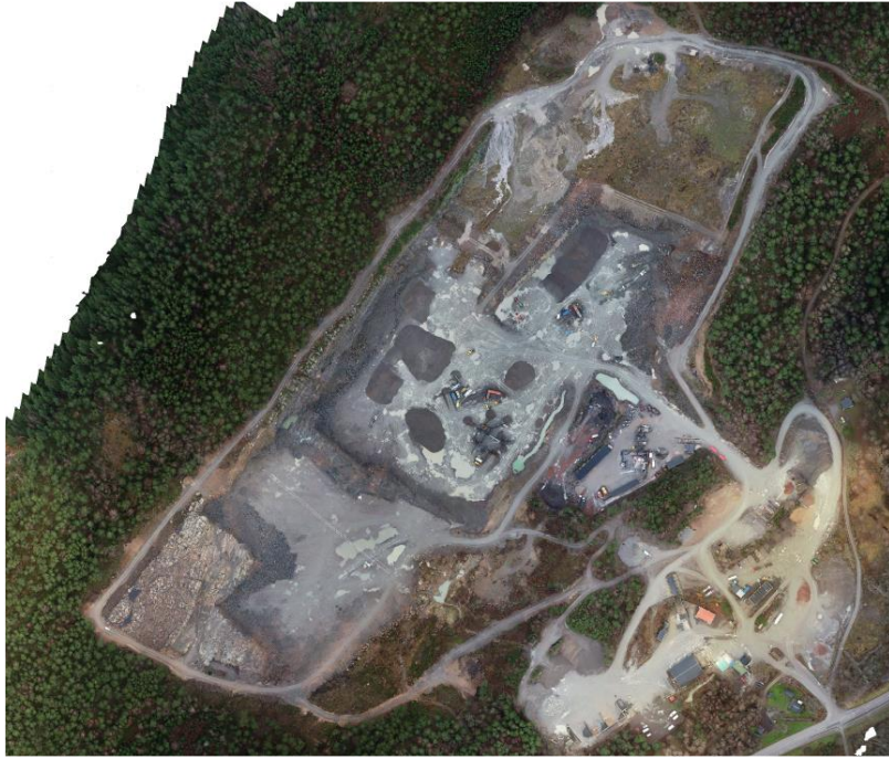
Figure 7: Overview of the quarry layout from December 2020 provided by NCC.
